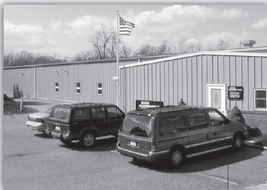
▲ 30,000 sq. ft. production facility in Elizabethville, Pa.
